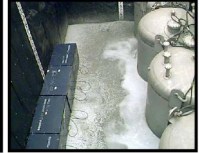
LLW Disposal Grouted in Vault
